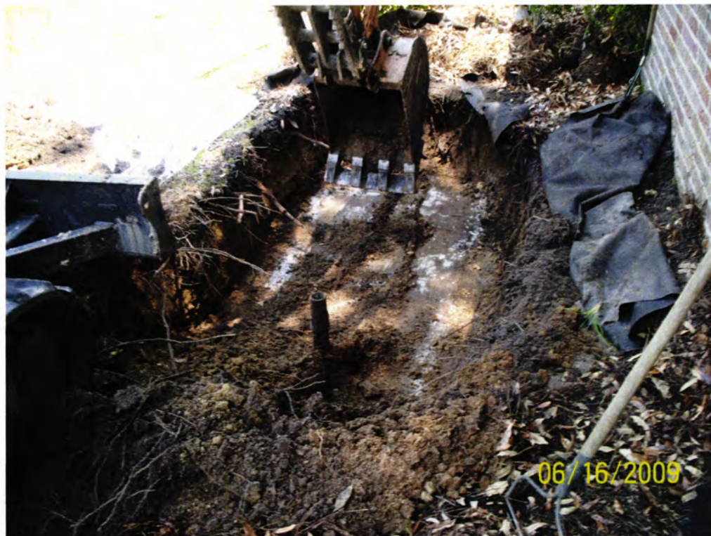
Picture 2: UST 1110Iris during excavation.
